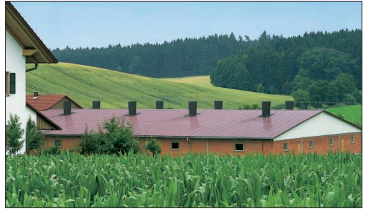
View on the same house from the outside
