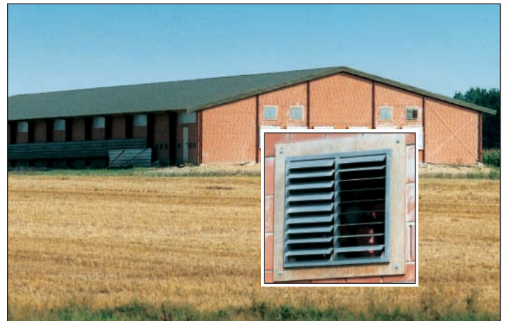
Use of wall fans
