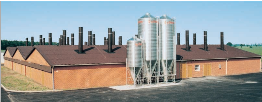
Decentralized exhaust air guiding
