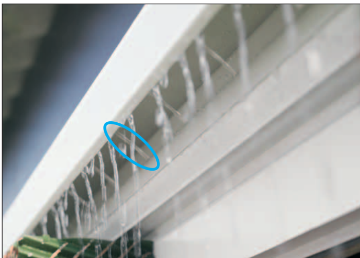
Top profile with perforated pipe and deflector for an even distribution of water along the pads
